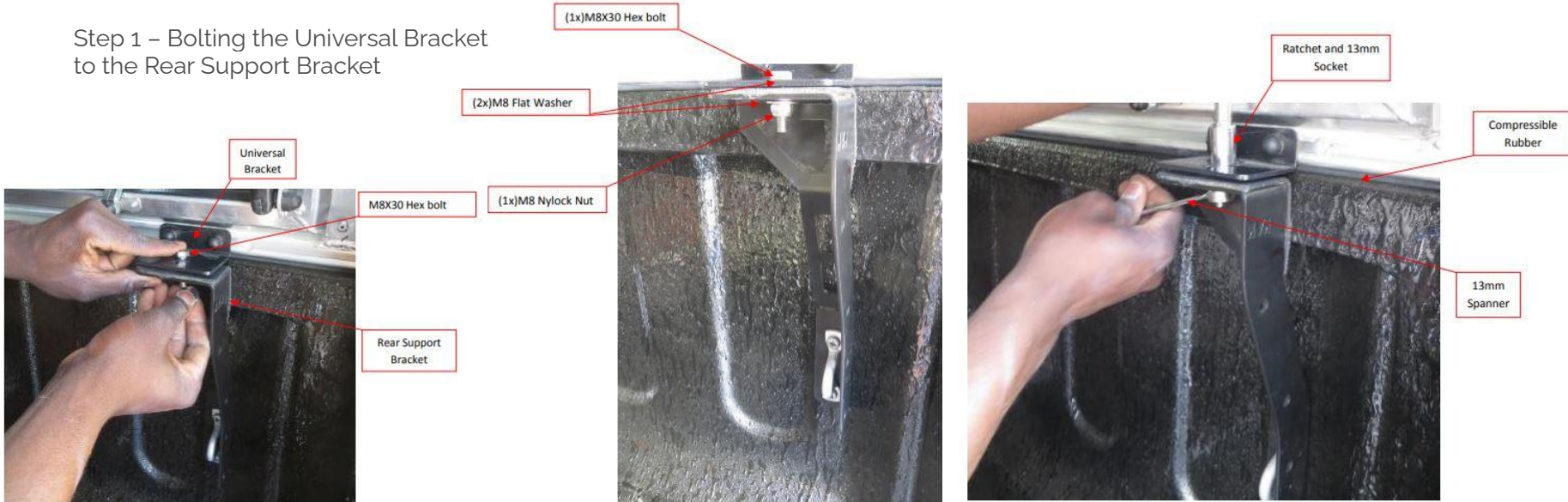
Figure 15: Inserting the Bolt for the Universal to Rear Support Bracket
